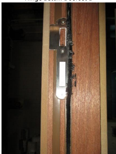
-Strike plate detail. Doorset B-
