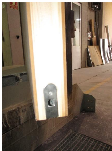
-Threshold drop seal detail-
