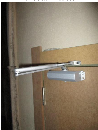
-Door closer detail. Doorset A-
