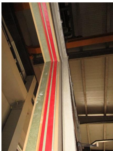
-Frame detail. Doorset A-
