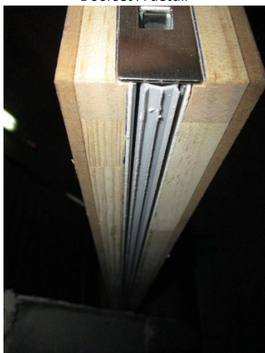
-Threshold drop seal detail.- Doorset A-
