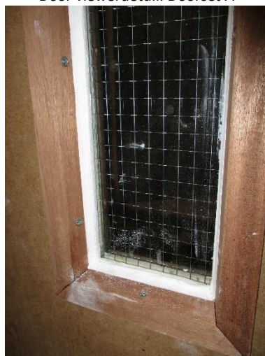
-Glass and moulding detail. Doorset B-
