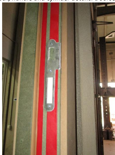
-Strike plate detail. Doorset A-
