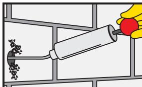
The drill hole must be cleaned with a blow pump or by compressed air, starting from the bottom of the hole. (at least 2x)
